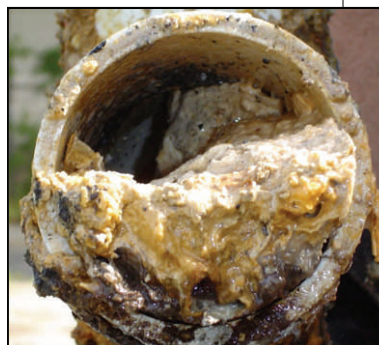
Typical Sewer Pipe Clogged with Fat, Oils, and Grease
