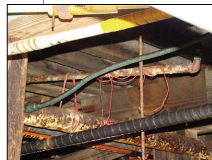
Wharf I Corroded Branch Line and Missing Hanger
